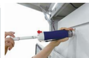
Checking filter saturation
